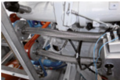
Stainless steel hose in a combined heat and power plant with swivel flanges
