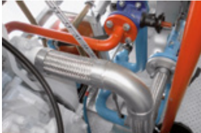
Stainless steel hose in a combined heat and power plant with 90° bend and swivel flanges
